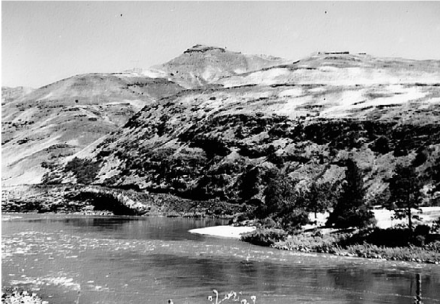
August 1953. Photograph of the right abutment for Brownlee Dam (photograph by F.R. McCormick). An open, scattered stand of pines are growing on a low river terrace/alluvial fan, with sandbar willow along portions of the river's edge. The slopes are moderate to steep, and substrates range from fines to cobble and bedrock. Sunflower is visible in the foreground, suggesting recent disturbance of portions of the site.
