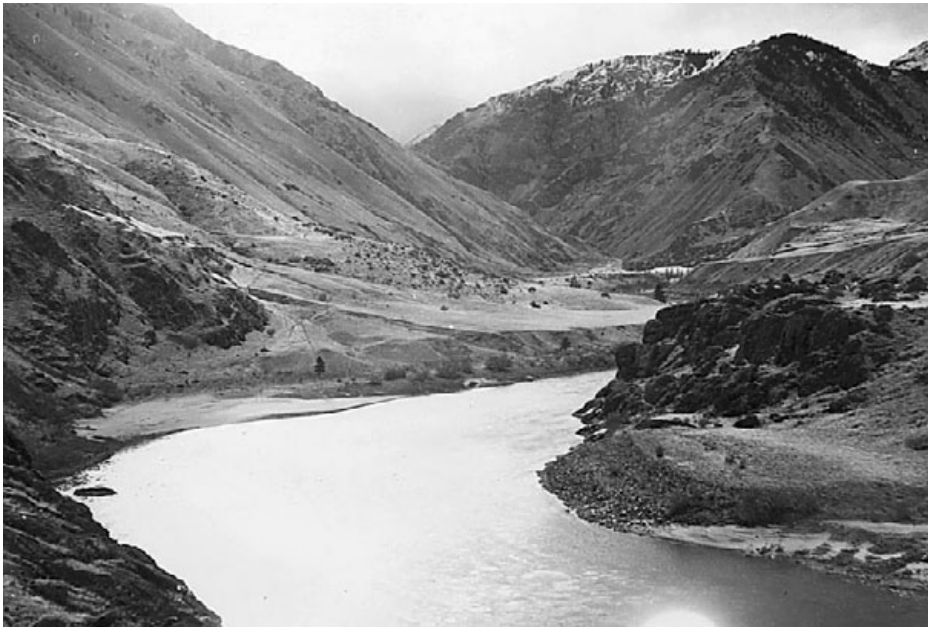
December 1953. Photograph of Johnson Bar showing a widely scattered riparian fringe of hackberry and channel-margin sandbars (photograph by F.R. McCormick). The broad, sloping terraces adjacent to the river are deposits related to the Bonneville Flood (14,500 years ago). Riverbanks consist of fines to cobble and bedrock.
