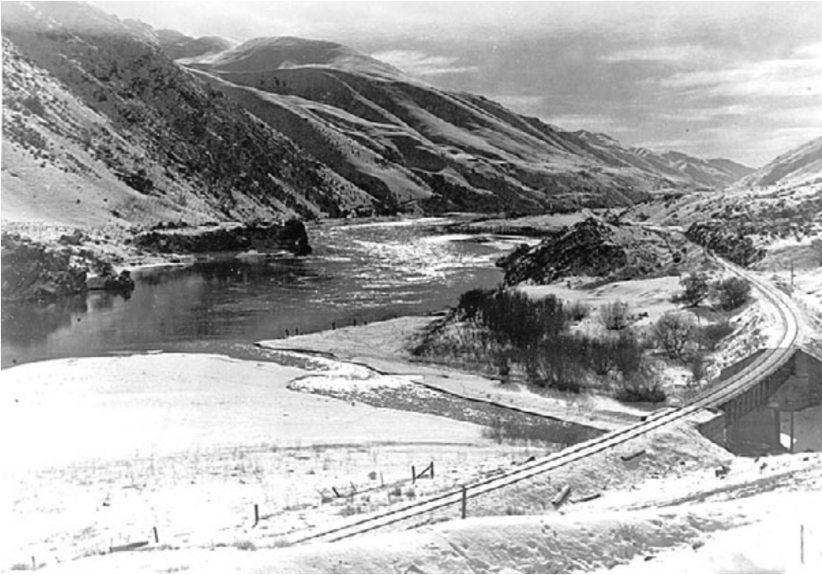
1946. Winter photograph of the Powder River confluence with the Snake River (photograph by P. Basche). Scattered hackberry and sandbar willows are visible along the riverbanks. Fine sands are abundant in this confluence zone, and most of the visible sandbar is barren. Adjacent upland slopes range from moderate to steep.
