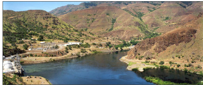
Fig. 12. Power-generating facilities at Oxbow Dam (lower left).
