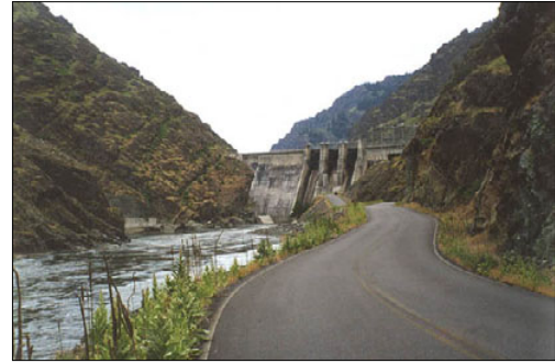
View from north looking south
