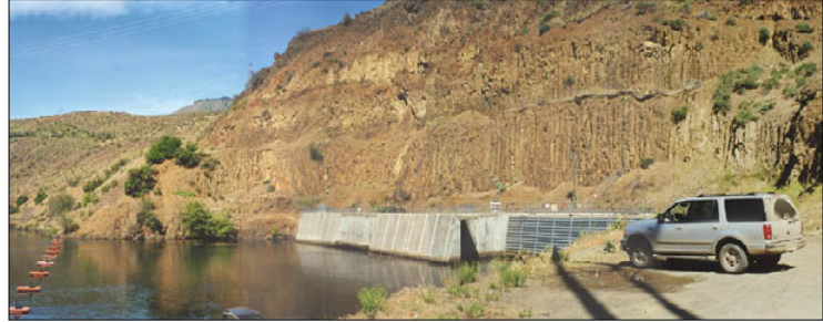
Oxbow Dam intake structure
