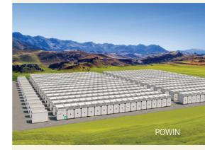
Although batteries don't generate electricity, they can store power generated during periods of lower use and deliver it when customers need it. A 40-MW battery array can power more than 13,000 average homes for four hours during periods of peak use, and more when energy demand is lower. The batteries can be completely recharged in about four hours, depending on their energy source.
