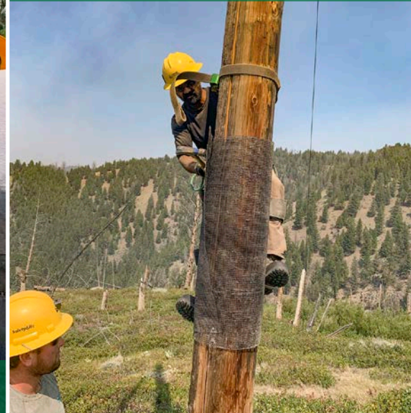
In areas of high fire risk, Idaho Power wraps some wood poles with fire-resistant mesh to protect them from wildfire.
