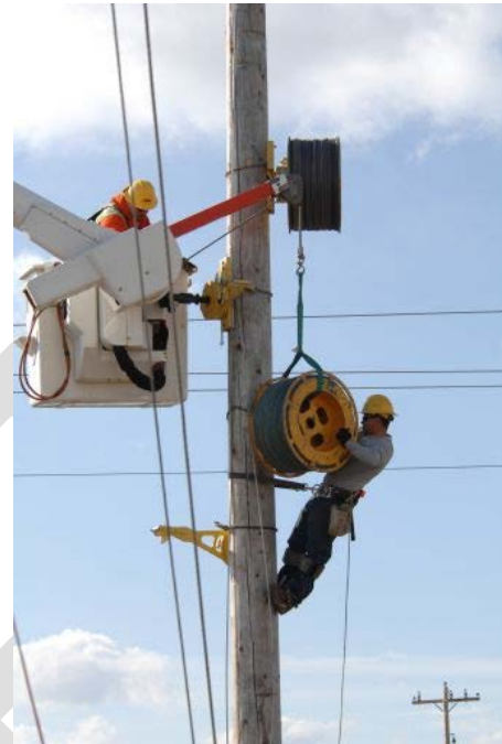
Idaho Power linemen install upgrades.
