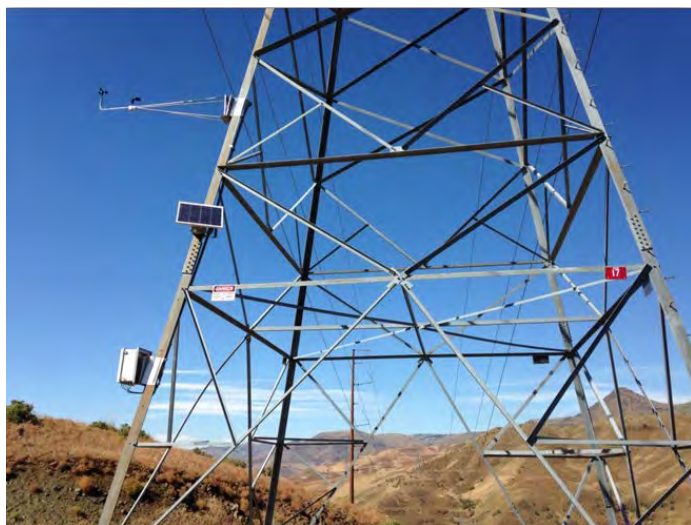
Figure 2. Dynamic line capacity equipment installed in Hells Canyon
