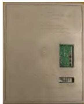
Figure 2. Aclara Load Control Transponder (LCT)
