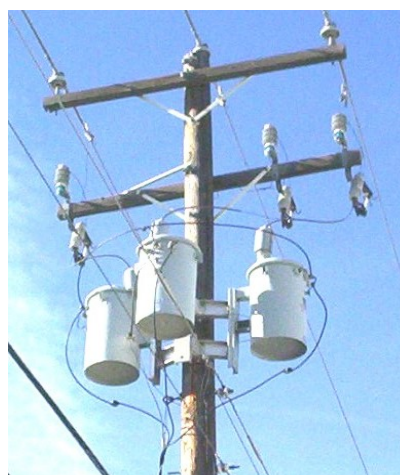
3-Ø Overhead Transformers
