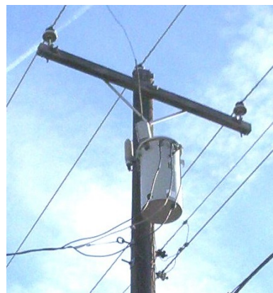
1-Ø Overhead Transformer
