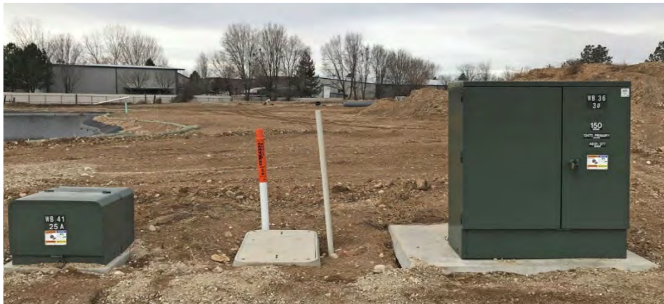
Figure 6 Single-phase and Three-phase Pad-mounted Transformers
