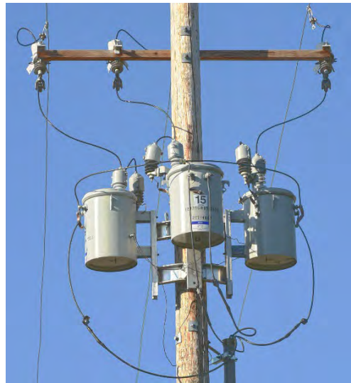
Figure 5 Three-phase Overhead Transformers
