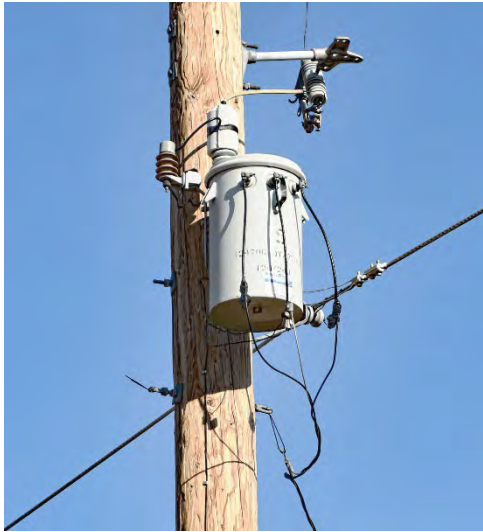
Figure 4 Single-phase Overhead
