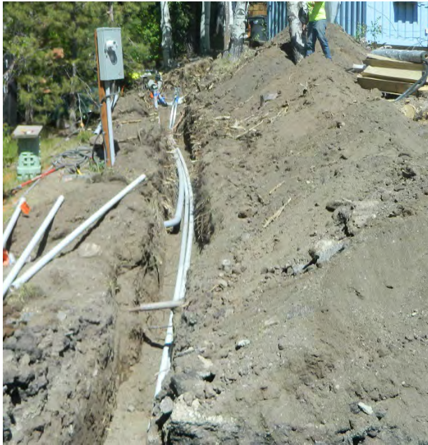
Example photo showing an unapproved trench with spoils too close to the edge, no conduit separation, and inadequate depth.
