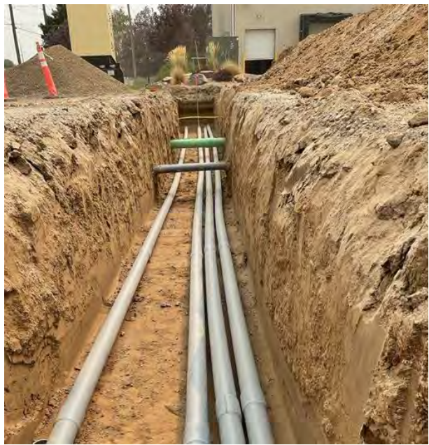
Example photo showing an approved trench with spoils 2 feet from the edge, proper conduit separation, and adequate depth.
