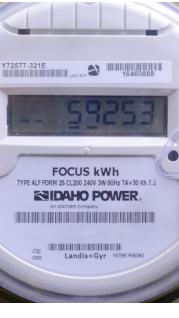
The Focus meter shows energy flow with a dashed line below the number showing energy usage or peak demand. When the dashes move left to right, you are using energy from Idaho Power. For customers with solar panels, right-to-left movement means you're sending energy back.
