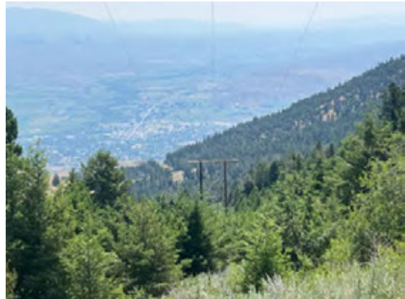
Figure 13 Salmon transmission line corridor pre-treatment (2025)
