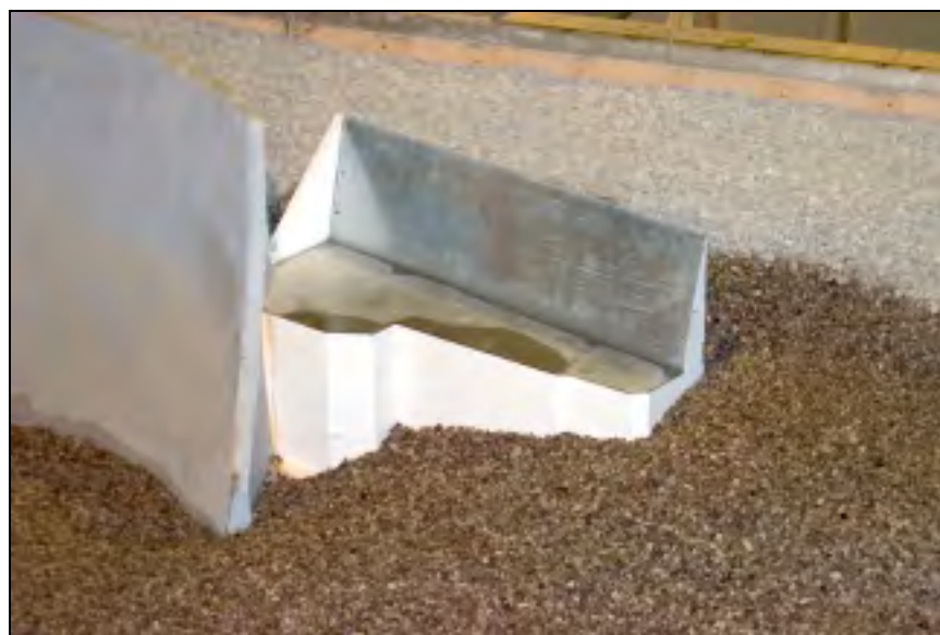
Figure 4.37. Fish ladder entrance scour after 40 kcfs per crest gate
