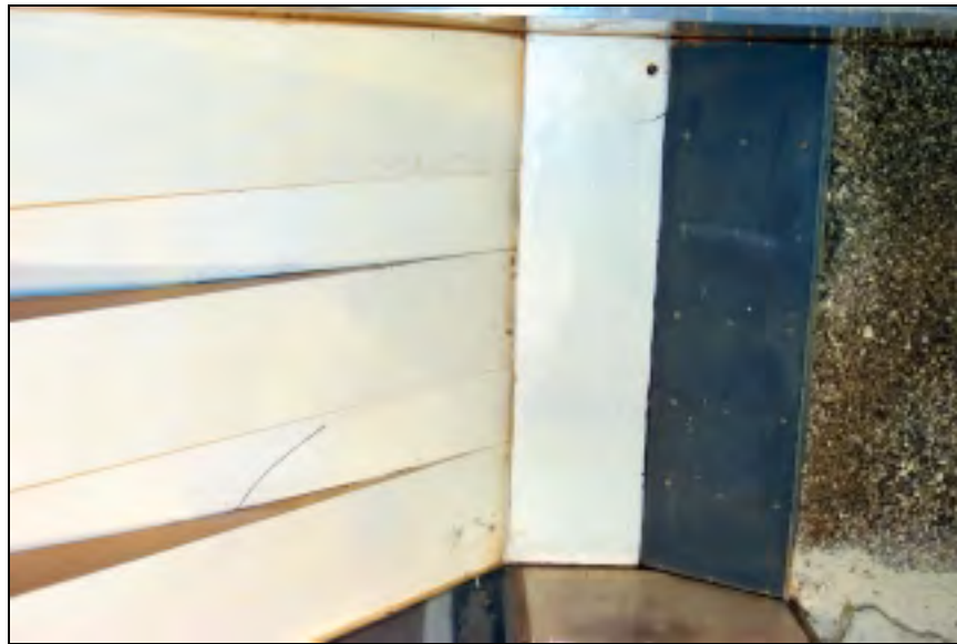
Figure 4.56. Clean apron after design discharge
