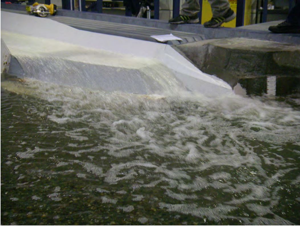
Photo 6.2.15 Deflector 17, 20,000 cfs, Low Tailwater, 2-Bay Operation
