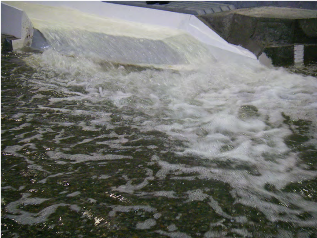
Photo 6.2.14 Deflector 16, 40,000 cfs, Low Tailwater, 2-Bay Operation
