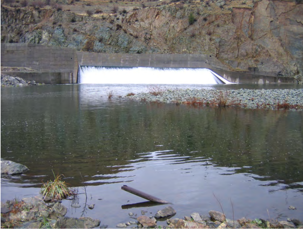
Photo 1.2 Oregon spillway operating at 100 cfs.
