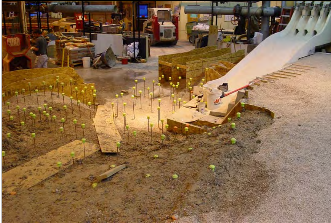
Figure 2-11. Photograph of bathymetric templates and grade stakes during construction
