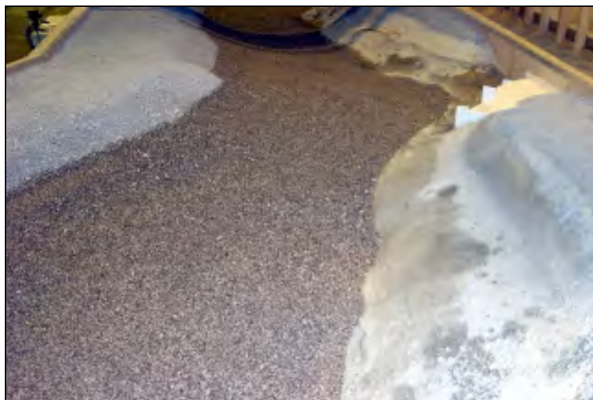
Figure 4.22. Looking downstream after 13.3 kcfs per crest gate
