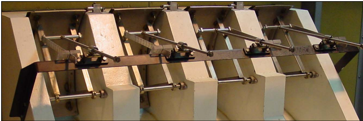
Figure 2-8. Photograph of the upper spillway gates
