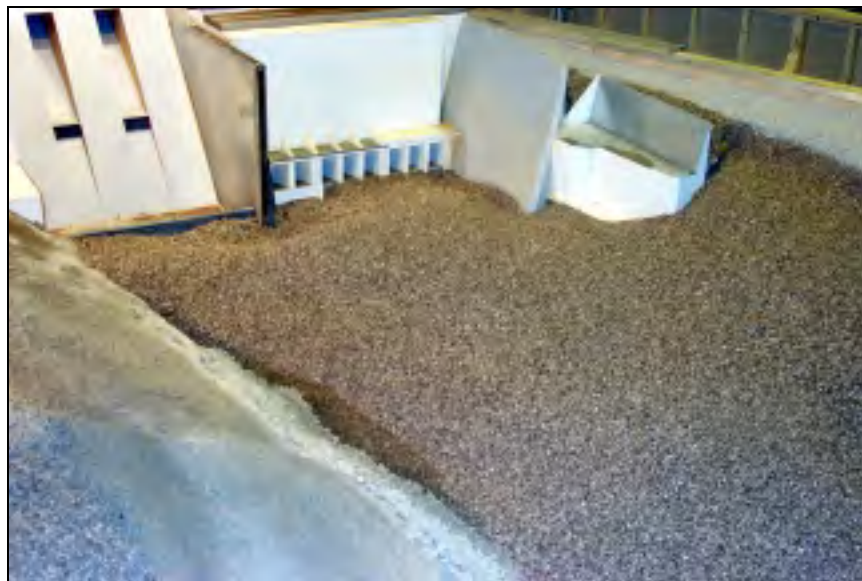
Figure 4.42. Fish ladder entrance scour after 50 kcfs per crest gate
