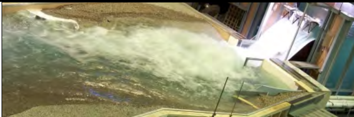
Figure 4.54. Panoramic view of spillway and stilling basin
