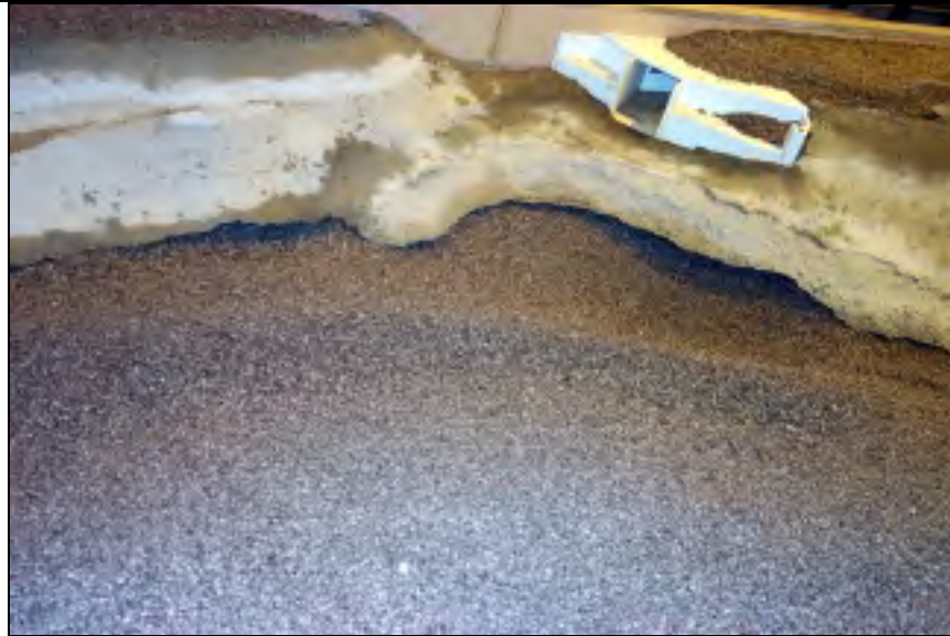
Figure 4.70. Scour hole near diversion tunnel outlet
