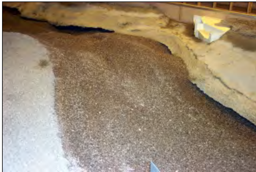
Figure 4.49. Downstream erosion after 67 kcfs per crest gate
