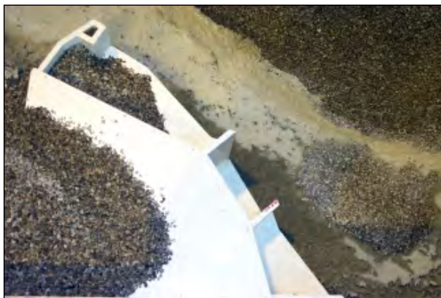
Figure 4.61. Rock deposits on bedrock and diversion tunnel structure
