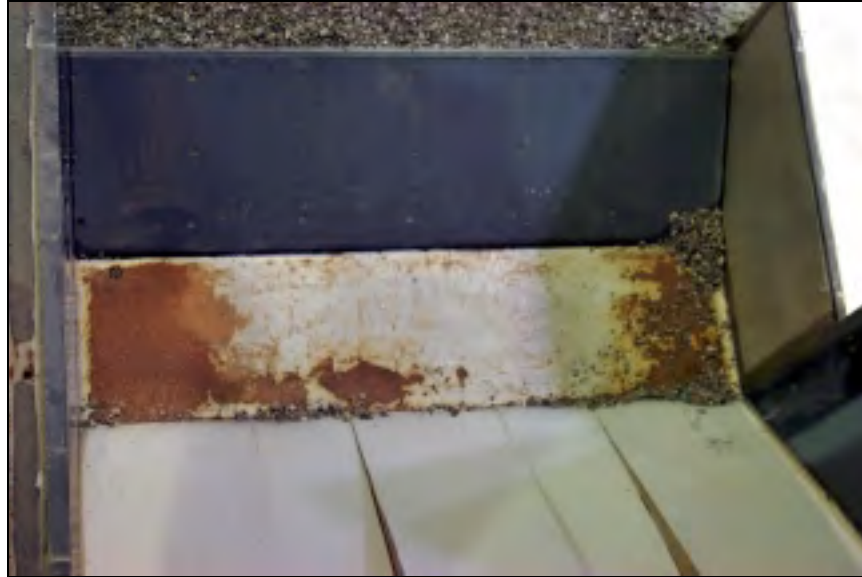
Figure 4.67. Material on apron after design discharge with deflectors
