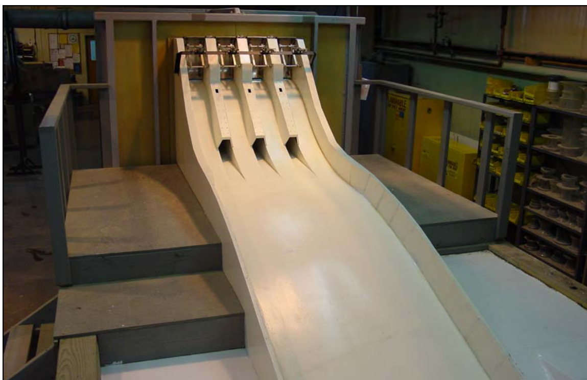
Figure 2-6. Photograph of the completed spillway
