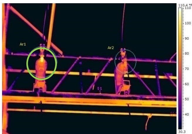
Figure 3.5 Infrared image of substation disconnects
