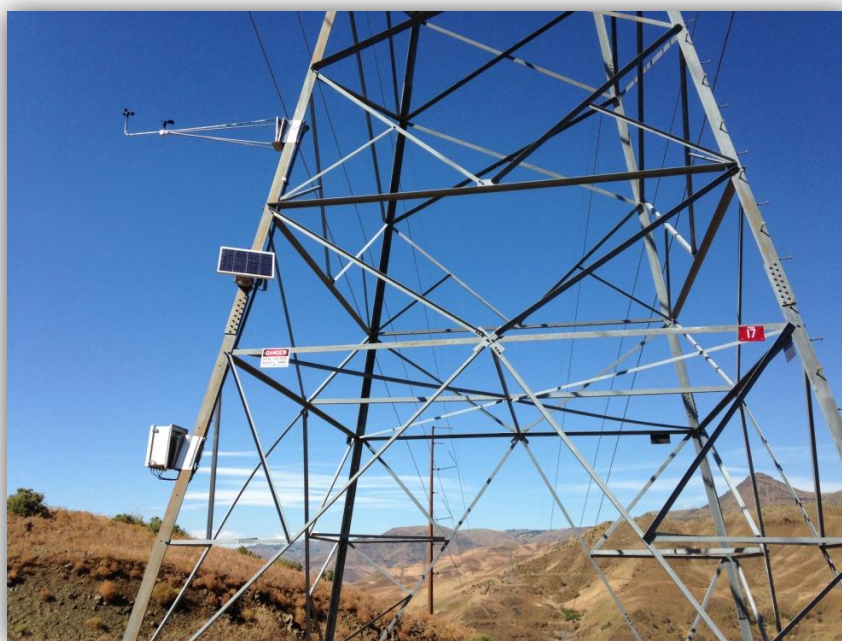
Figure 2. Dynamic Line Rating Equipment Installed in Hells Canyon
