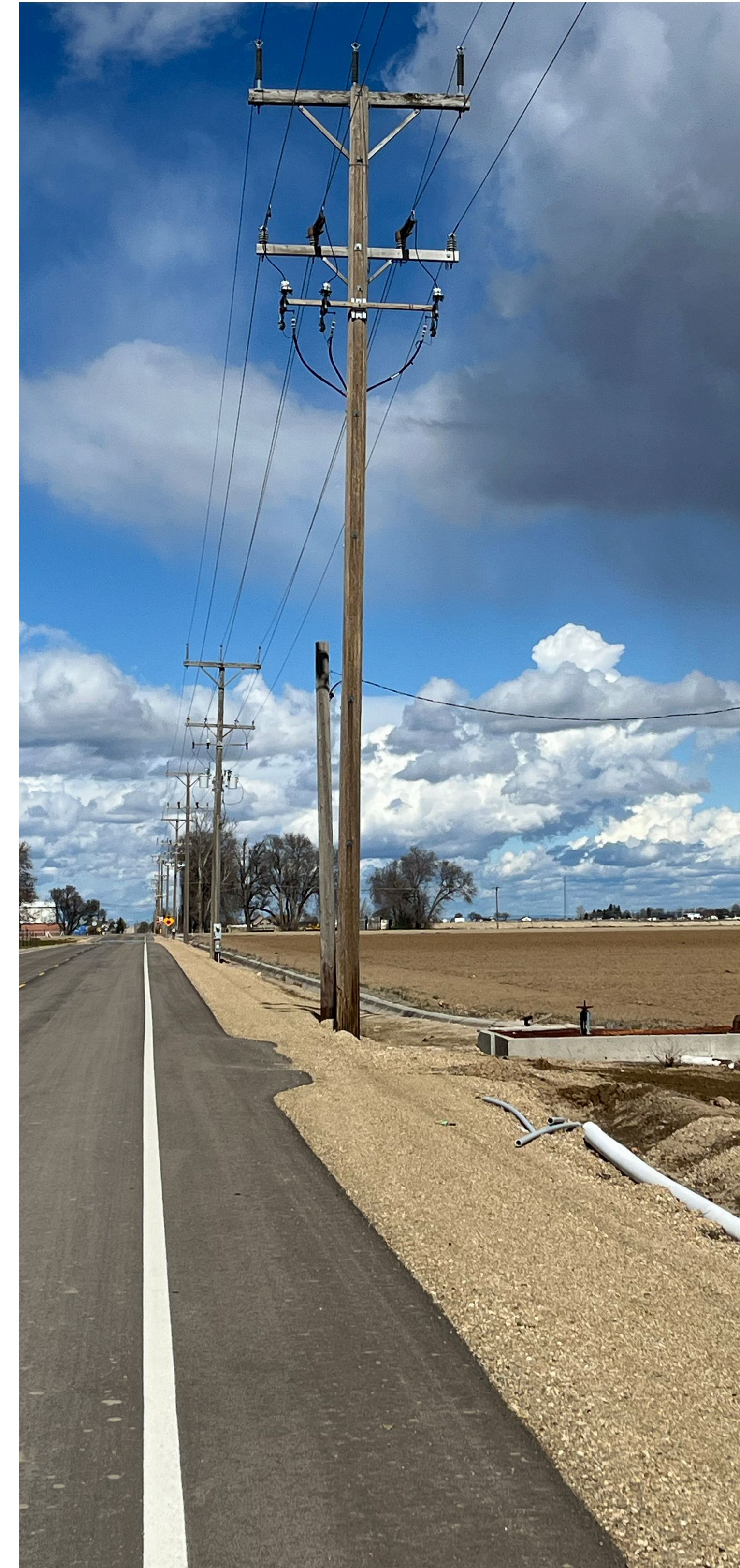
Existing wood pole in project area.
