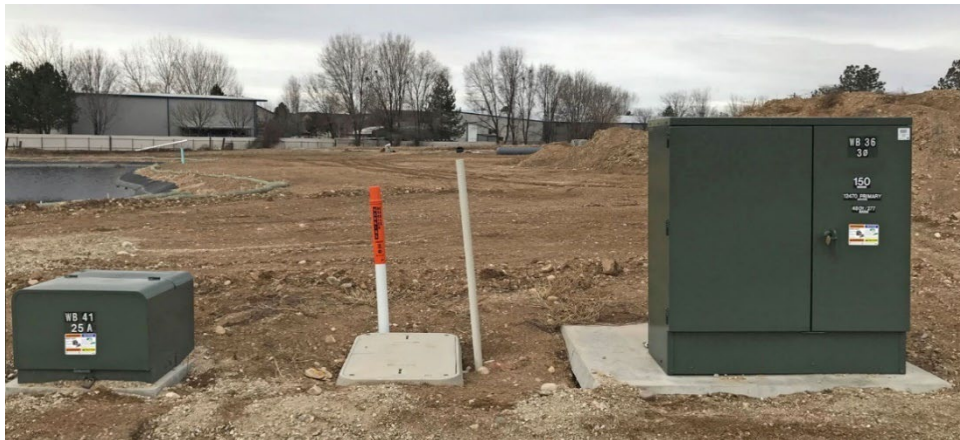
Figure 6 Single-phase and Three-phase Padmounted Transformers
